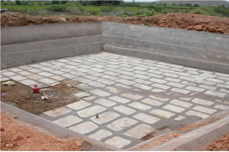
Fig. Farm Pond Lined with Fire Bricks
