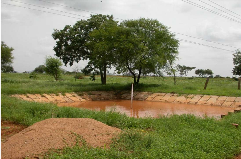
Fig. Farm Pond Lined with Kadapa Slabs
