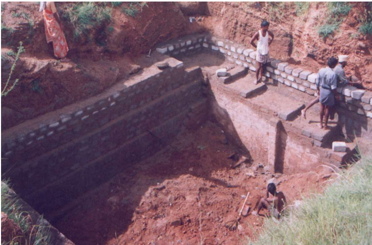
Fig . Farm Pond lined with Cement Bricks
